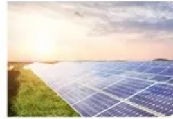
Energy Storage System
