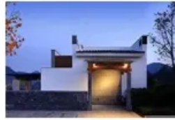
Household Energy Storage
