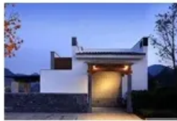
Household Energy Storage
