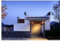
Household Energy Storage
