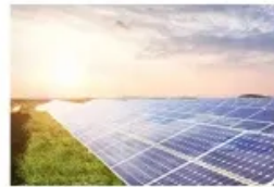
Energy Storage System
